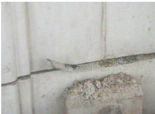
**Figure 4. Titanium Ribbon Mesh installation in mortar joint.**
