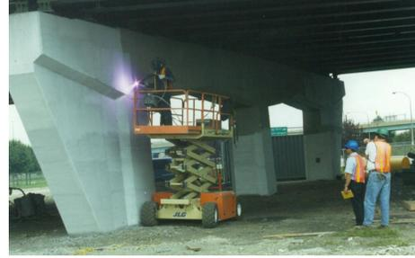
**Figure 6. Arc-spray application of sacrificial Aluminum-Zinc-Indium**
