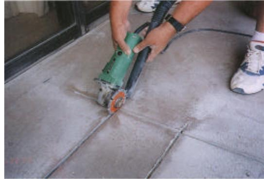
**Figure V. Slotted system installation on the top side of a condominium balcony in Florida.**
