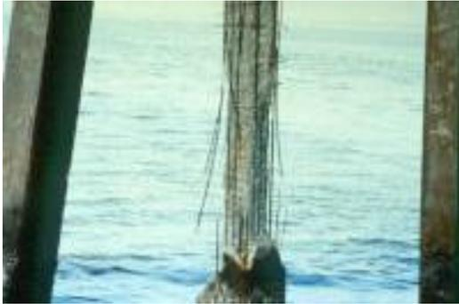
**Figure II. Previously repaired concrete bridge pile in a marine environment, Florida.**
