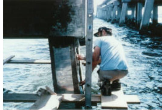
**Figure VIII. Zinc adhesive anode being applied to a bridge pier in Florida.**
