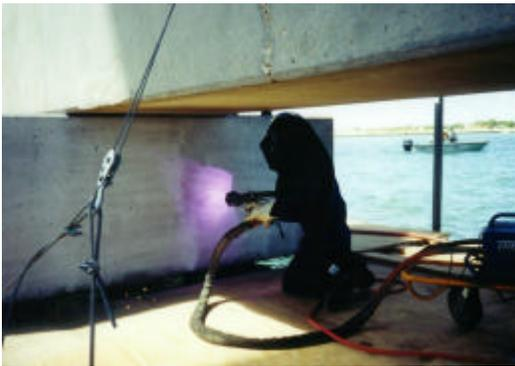
**Figure VII. Arc spray application of galvanic Al-Zn-In to a bridge pier in Texas.**
