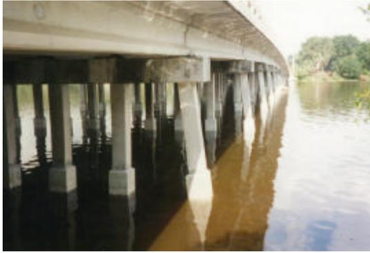
**Figure IV. Integral pile jacket system on bridge piles in Florida.**
