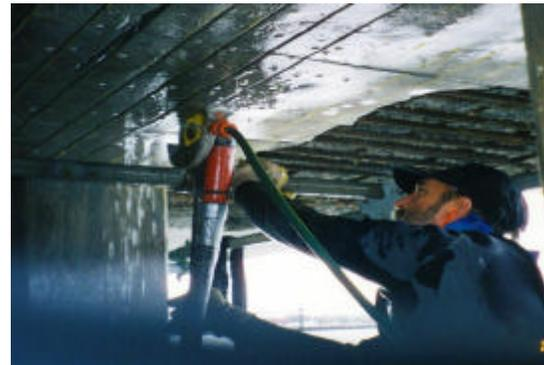
**Figure VI. Slotted system installation on the underside of a wharf terminal in Australia.**
