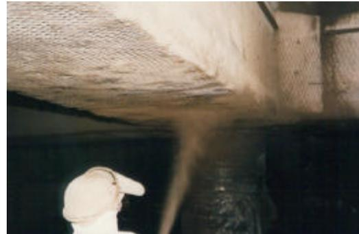
**Figure III. Titanium anode mesh encapsulation with shotcrete, Hong Kong container berth.**
